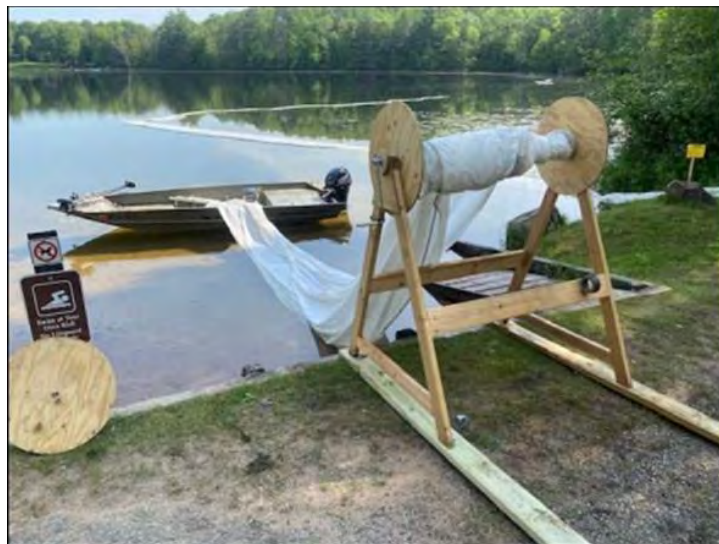
Figure 52: Limno-curtain material on a roll before installation (photo from Marinette Co. LWCD)
